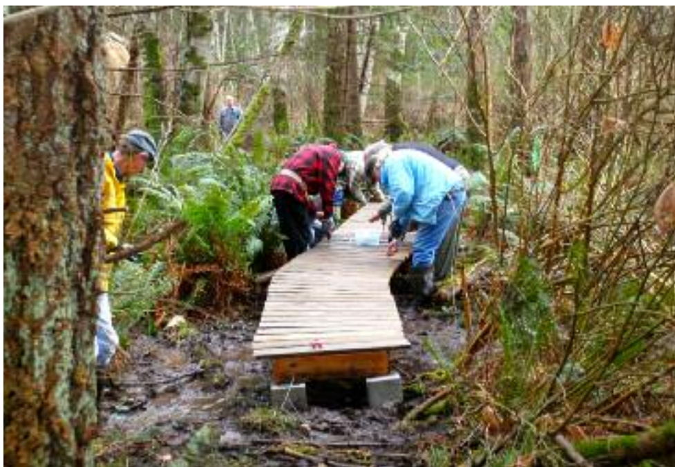
A GaLTT work-party constructs a boardwalk on the swampy section of Sally Robinson's licensed trail between Cooper and Islands View. [Photo by Barb Hague]
